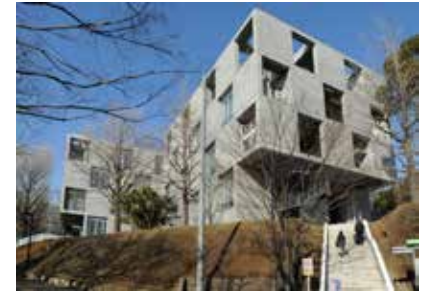
Midorigaoka-6th Building Under Construction, design S. Okuyama ; structure T. Takeuchi
