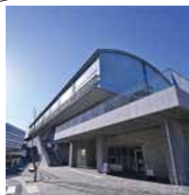
West 5th & 6th Building. 2023, design S. Nasu, T. Shiozaki structure T. Takeuchi
