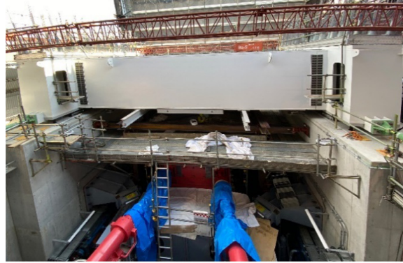
(b) Installed reaction beam on elastomeric isolator bearings
