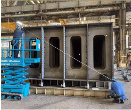
(a) Fabrication of reaction beam
