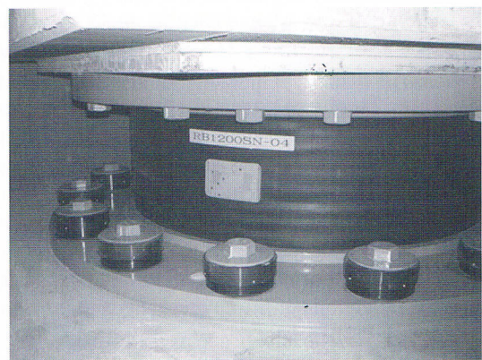
Figure 12. Setting of spring washer.
